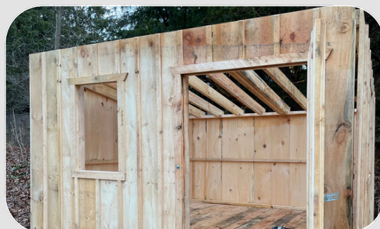
March: adding the roof
