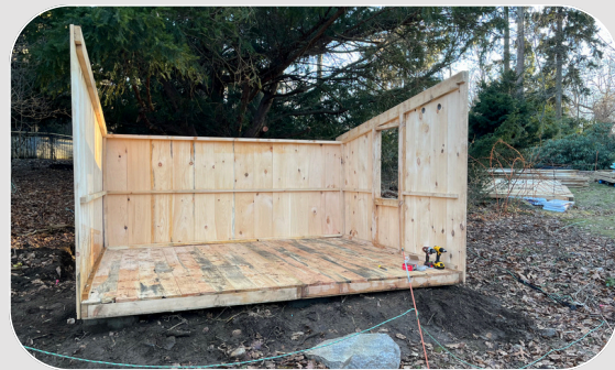
February: building the walls
