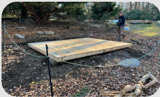
January: building the foundation
